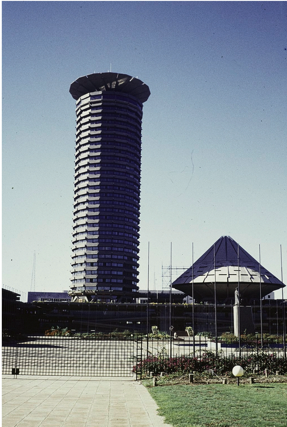
Fig. 3. Reverse slide of Kenyatta International Conference Center, Nairobi. Photograph taken by Aart Rietveld, 1975.
