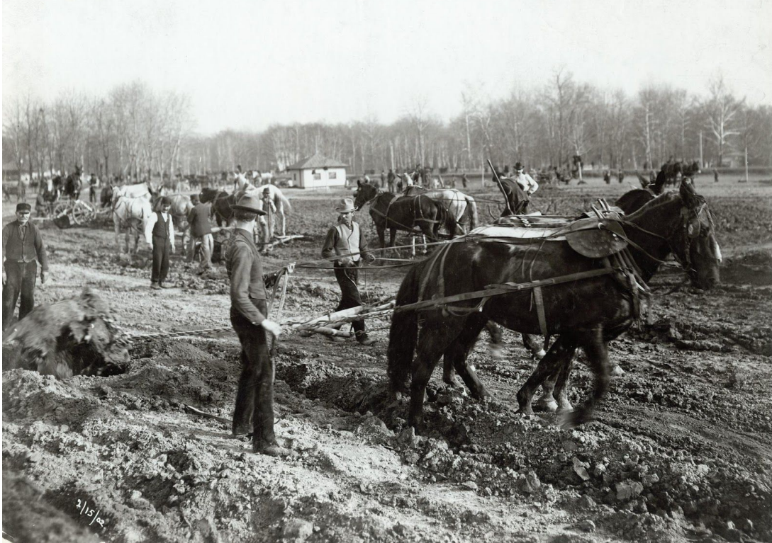
World's Fair Construction, 1902. Courtesy of the Missouri Historical Society, St. Louis, N15483.
