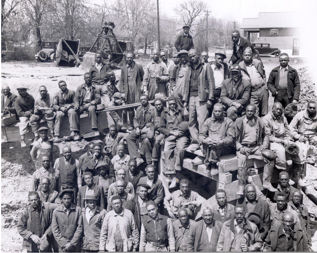
Works Progress Administration (WPA) workers constructing an enclosure for the river in University City, 1940. Courtesy of the Missouri Historical Society, St. Louis, N01825.
