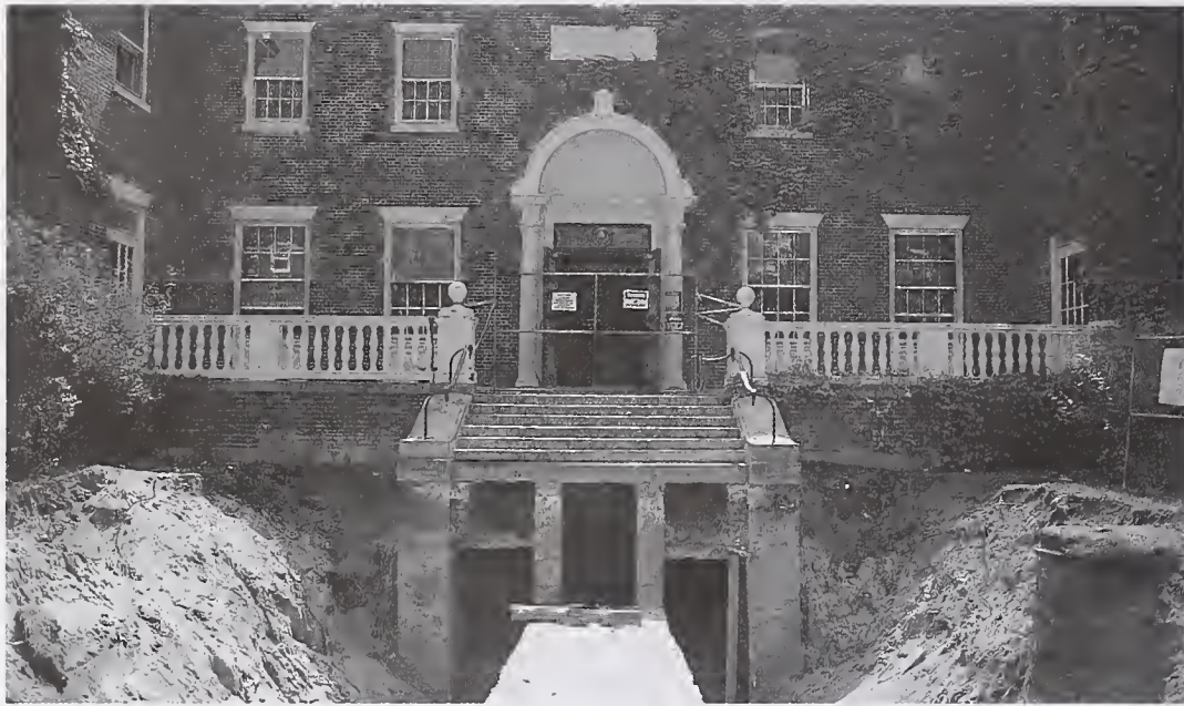
Moulton Union renovations in progress, summer 1995.
