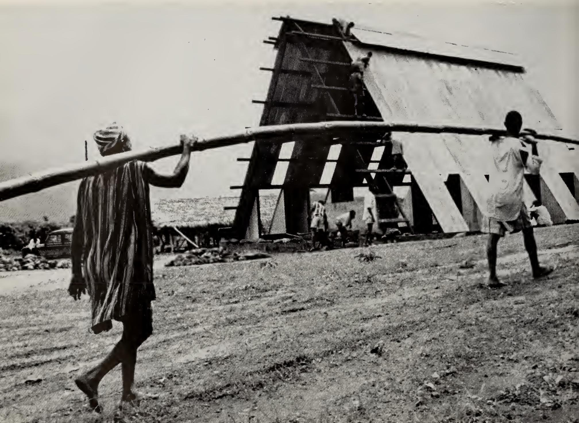
**Sierra Leone needed a structure that was inexpensive, comfortable, easy to erect—and able to withstand wind, termites, and heat. The answer: an A-frame designed by VITA members in North Carolina and New Jersey.**
