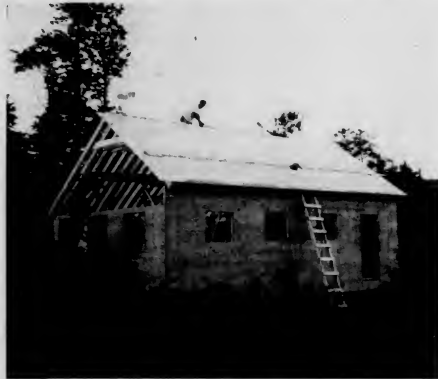
An Outing Club member is busy constructing the cabin.
