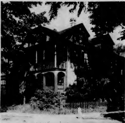
The Chamberlain House as it stands today on Maine Street.
