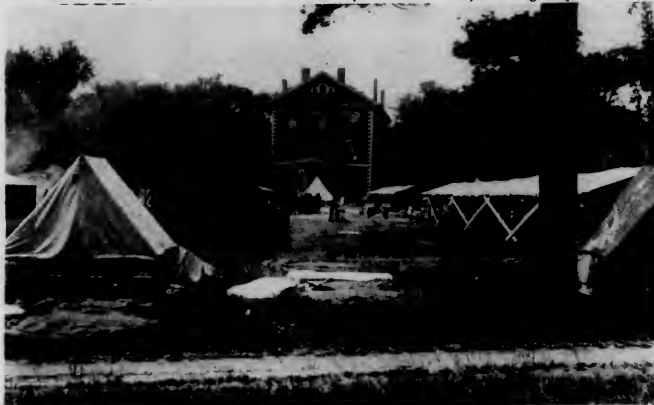
Photo courtesy of the Pejepscot Historical Society. Mess tents were set up where Sills is now located.
